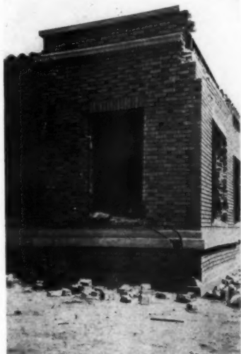
FIG. 15. DAMAGE CAUSED TO CORNER OF COMMERCIAL BUILDING BY DIAGONAL TRUSSES
